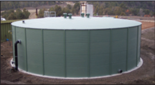
GALAXY® 194,000 gallon water tank installed in La Plata County Colorado. Stores well water and Brine as part of a commercial application.
